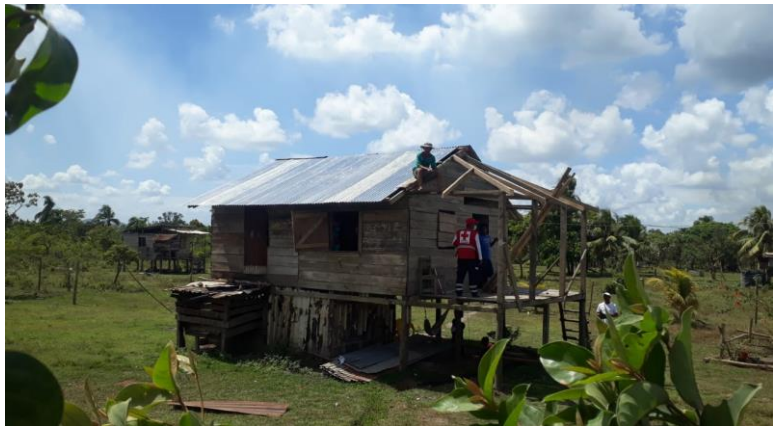
Shelter component promoter assisting and monitoring the reconstruction of beneficiaries' homes, 10 May 2021. Source: NRC
